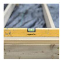
To check that your base is level, place a straight edged piece of timber across the length of the base and place a
