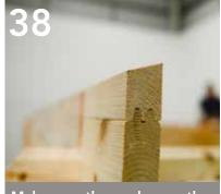
Make sure the angles run the correct way to define the slope of the roof.
