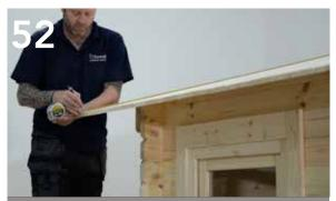
Transfer this measurement to the end board on either side of the cabin.
