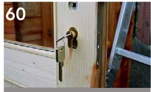
Firstly locate the Euro Cylinder into the mortice lock. Use the keys and turn slightly allowing it to fit in.
