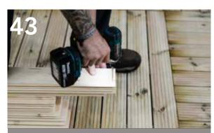
Pre-drill two holes in the top of each roof board. Do this on one end of each roof board only, this is the end that will attach to the middle rafter.
