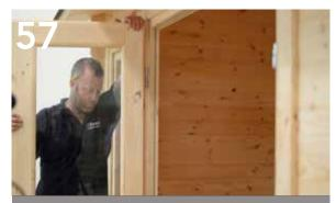
Line up the male and female parts of each hinge and lower the doors into place.
