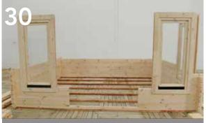
Build the cabin up to about 8 logs high then slide each window frame over the logs. This will help act as a guide for all additional logs.
