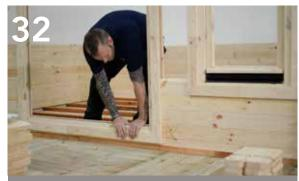
Make sure the door and window frames are pushed down fully.
