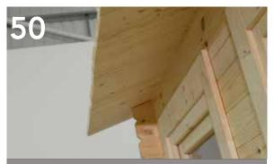
When all the roof boards have been installed the roof board edges which overhang the front and rear of the cabin will need to be trimmed flush.
