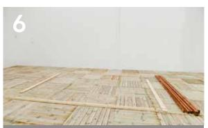
Locate the floor bearers, the two half logs and two of the full wall logs (refer to the instructions if needed). Take these to the site of installation and lay out as shown.
