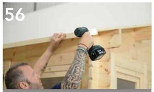
Pre-drill both ends of each strip and once in the middle (three screws per section). Before fixing into the end grain of the roof boards, ensure the top of the end grain protection strip is flush with the top of the roof boards and the end of the strip is flush with the outside edge of the end roof board.
