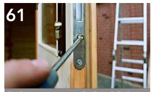
Fit the screw to secure the Euro Cylinder. If you peer through the screw hole you should be able to see the threaded hole in the Euro Cylinder, in which it has to locate. If not wiggle it around until you do.
