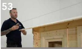
Apply a chalk line on these two measurement points and mark a line across the entire width of the cabin.
