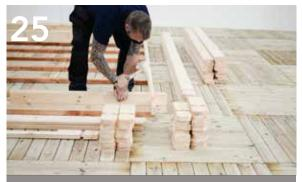
Start building the cabin walls by securing a full log to each of the half logs.
