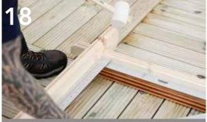
Ensure the base is square by applying a builder's square to each corner and tapping into position. Measure across each diagonal, ensuring they all measure the same distance. Make adjustments as necessary to bring the base into a perfect square.
