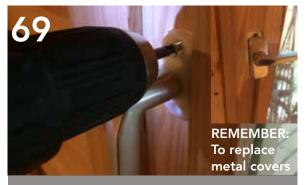
Fix in place using the flat head screws located in the fixing pack.
