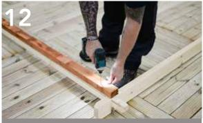
Make sure each end of the floor bearer is lined up flush with the outside edge of the full wall logs then pre-drill a hole ready to fix the bearer and log together.
