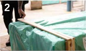
In order to unpack your cabin first unpack the doors and windows, and felt/shingles which have been stacked on top of the main cabin. Carefully cut the strapping and remove the packing timbers. Then remove the packaging from around the cabin. Take care when removing the packaging as it is stapled to the cabin logs to keep it in place during transit.
