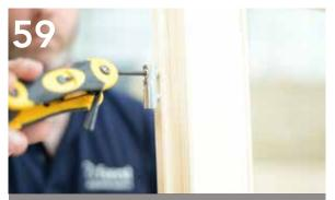
If the doors need adjusting, lift them back off the hinges and use an Allen Key to adjust each hinge accordingly.
