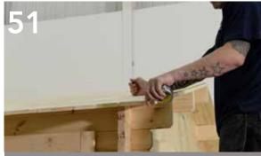
To do this, locate the shortest board and measure the distance between the apex point of the roof and the end of the board.
