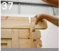
Fit the front and rear roof edge support logs.
