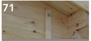
Ensure each brace is fitted to the top rafter of the cabin on the front and back, and spans the apex and walls on each side. Mark out each hole and drill the necessary holes. Secure in place using the M10 bolts, washers, and nuts supplied with the fixing pack. Fit each storm brace to the outside of the cabin.
