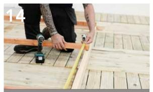
Make any final adjustments then pre-drill and secure each end of the bearer to the wall logs using screws.
