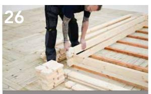
Interlock a side log over the front and back rear logs.
