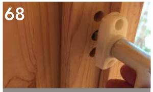
When fitting the window handles remove the metal cover and insert the handle into the three pre-drilled window holes.
