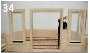
Using the window and door frame as a guide, continue to build the walls of the cabin up to roof height.
