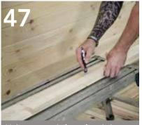
Using a straight edge join the joist marks together on the roof board by drawing a cutting line.
