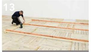
Continue to secure to the half log in the centre and other end of the floor bearer. Repeat for the other edge bearer. Position one of the floor bearers roughly in the center between the two edge bearers. Measure from the outer edge to the center of the middle bearer. Measure from the adjacent outer edge until the bearer is dead centre.
