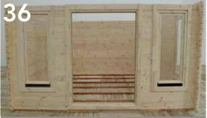
Once the front recessed log, rear full log and two side logs have been fitted you are ready to start constructing the framework for the roof.
