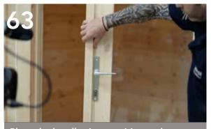
Place the handles into position and secure by tightening the small grub screw on the side of one handle.
