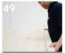
Place the cut down roof board into position. Pre-drill and screw once to each rafter.
