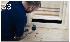
If needed, release some of the tension on the window and door frames by slightly loosening the frame screws. Once the internal part of the frame is fully in contact with the top of the log supporting it, re-tighten the screws.
