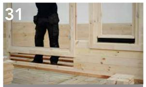
Slide the door frame over the logs and into position.
