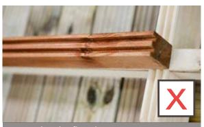
Do not lay the floor bearer on its narrowest edge otherwise the internal lip to support the floor boards won't be created.
