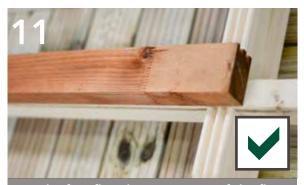
Lay the first floor bearer on top of the flat surface of the half log making sure the edges of the bearer line up flush with the outside edge of the half log. Also ensure the bearer is laid on its widest edge.
