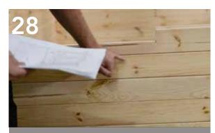
Build the logs up to window height. Referring to the instructions, note how many logs are needed to be installed before the window recess log is installed.
