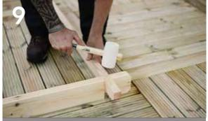
Before securing the logs together, ensure both the flat part of the half log and the grooves of the full log are face up.
