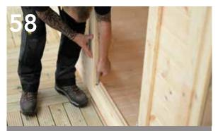
Ensure the shoot bolts located at the top and bottom of each door align with the shoot bolt holes located within the door frame.
