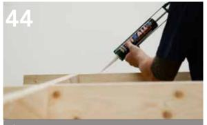
If applying adhesive, only apply enough to each rafter for three or four roof boards at a time as it's quick drying.
