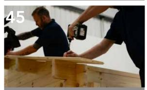
Place the edge of the first roof board flush with the edges of the rafters. Pre-drill and screw each roof board twice to each rafter working your way from one side of the cabin to the other.
