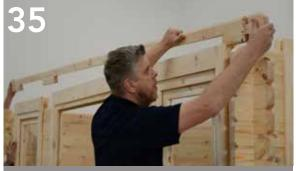
When installing the top recessed logs, as before, loosen the tension on the window and door frames to allow the logs to rest perfectly on top of the window and door frames.
