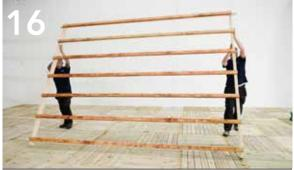
With the help of another person, lift the finished base at one end. Once the base is in a vertical position proceed to 'flip' it over so the bearers will end up resting directly on the floor.
