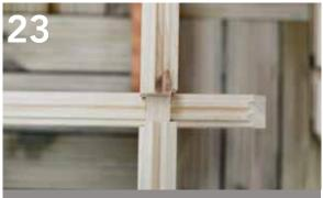
The joints should interlock tightly as shown. Note that the tongue of the logs should always be face up.
