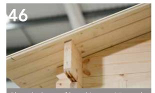
Place the last roof board into position and mark the position of each rafter edge on the underside of the board.
