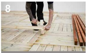
Using a white faced rubber mallet, connect the half log to the full log. Please ensure you strike the log on the inside of the joint, not on the outside where you risk snapping the end of the log off.
