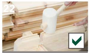
Please ensure a rubber mallet is used at all times when striking the logs. Always strike the logs on the inside of the joint.
