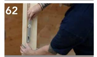
Place the door handle covers over the barrel lock and line the holes up.
