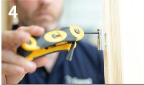
Using an Allen Key, turn the adjustment bolt anti-clockwise to push the door closer to the adjacent door, or turn it clockwise to pull the door back towards the door frame. Repeat with the bottom hinge as necessary.
