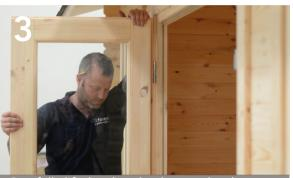
Carefully lift the door back onto the door frame hinge and check the adjustment. If further adjustment is required, lift the door back off the hinges and repeat the process as required.
