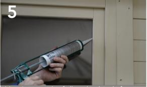
Most importantly of all apply a bead of silicone around the perimeter of the frame where it meets the glass.
