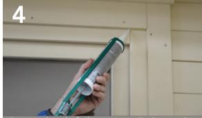
Ensure a bead of silicone is applied around the entire perimeter of the inner frame making contact with both edges of the frame to provide a seal.
