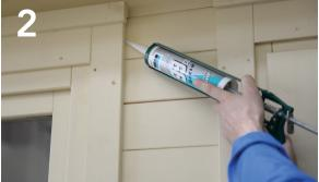
Seal around the outer perimeter of the frame where it meets the logs of the cabin. Always ensure the bead of silicone makes contact with the frame and cabin logs to provide a good seal.
