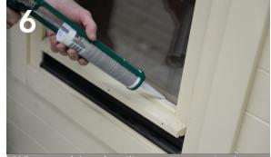
When applying the silicone try to maintain an even pressure on the applicator and use a smooth slow movement as you move the nozzle across the frame.
